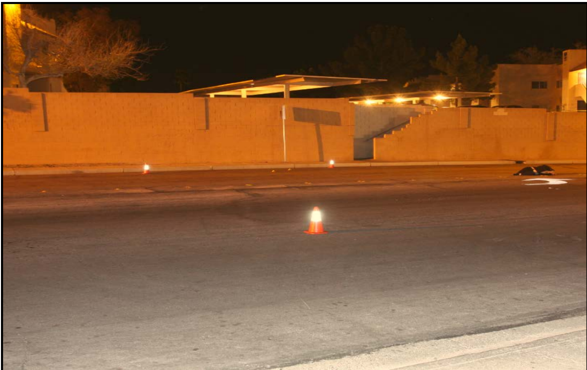
Block wall lining the North side of the scene
